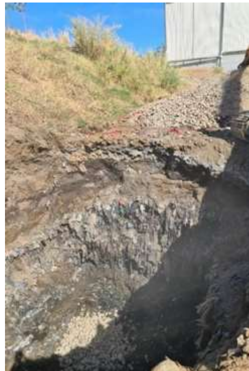
Photo N° 10: Trench T-4 located above the sanitary landfill cell. Trash
