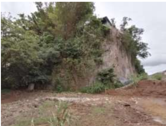
Photo N° 5: Detailed rock slope where the dike would end.
