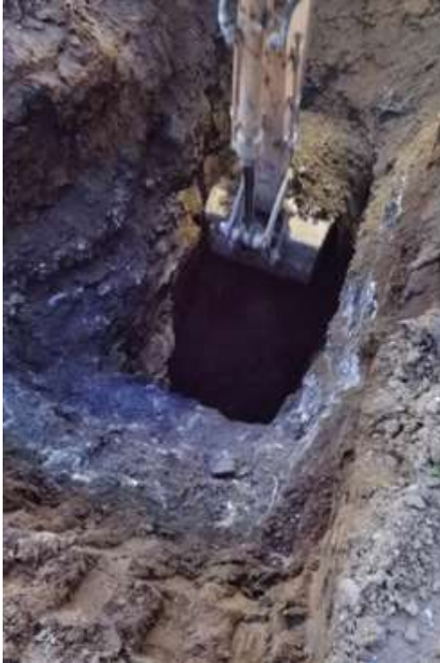
Photo N° 9: view of the T-3 survey, located on the road. 1.0 m layer of soil, then ballast. Compacted.
