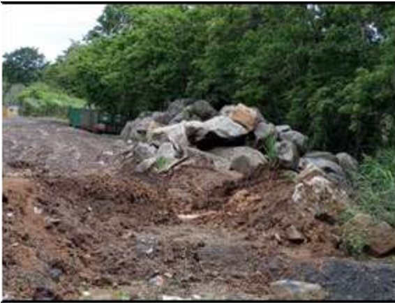
Photos N° 7 & 8: Details about rock blocks brought from another project in which the EBI is carrying out work, to form the closure dike.
