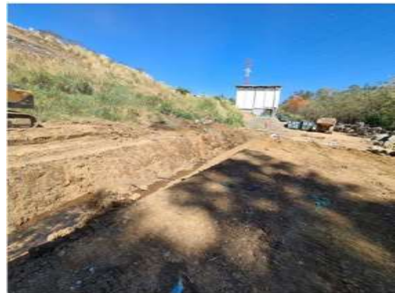
Photo N°12: Trench for a 12" pipe that passes under the closure dike.
