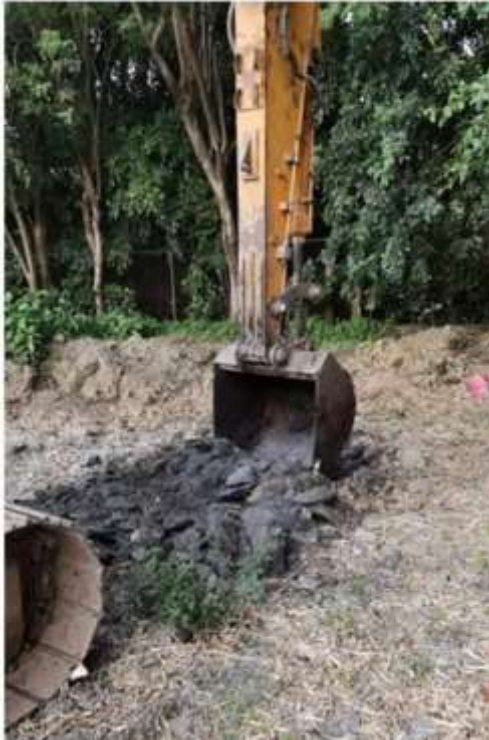
Photo N° 9: Trench T-1 near the cyclone mesh, property boundary. Rock material. Hard.
