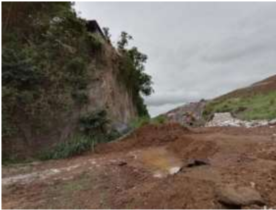
Photo N° 3: East zone of PTA La Uruka, where the closure dike will be built. On the left the rock slope would finish the dike.
