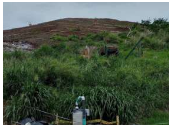
Photo N° 6: Internal road zone (beginning of dike).
