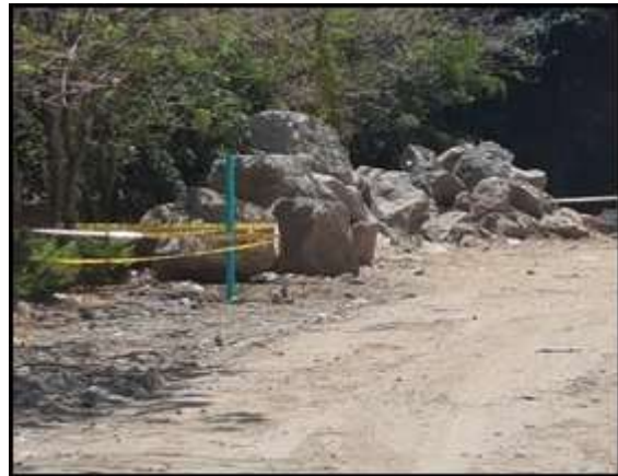
Photos N° 7 & 8: Details about rock blocks brought from another project in which the EBI is carrying out work, to form the closure dike.
