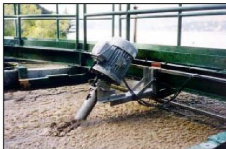
Typical TORNADO Aerator Installation.
