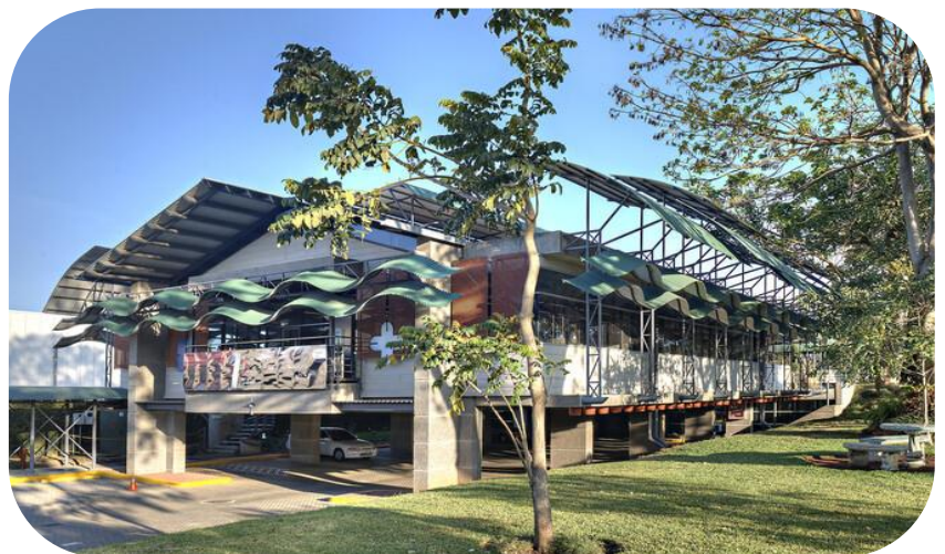
BATCCA Caribbean-Central America Office Building
