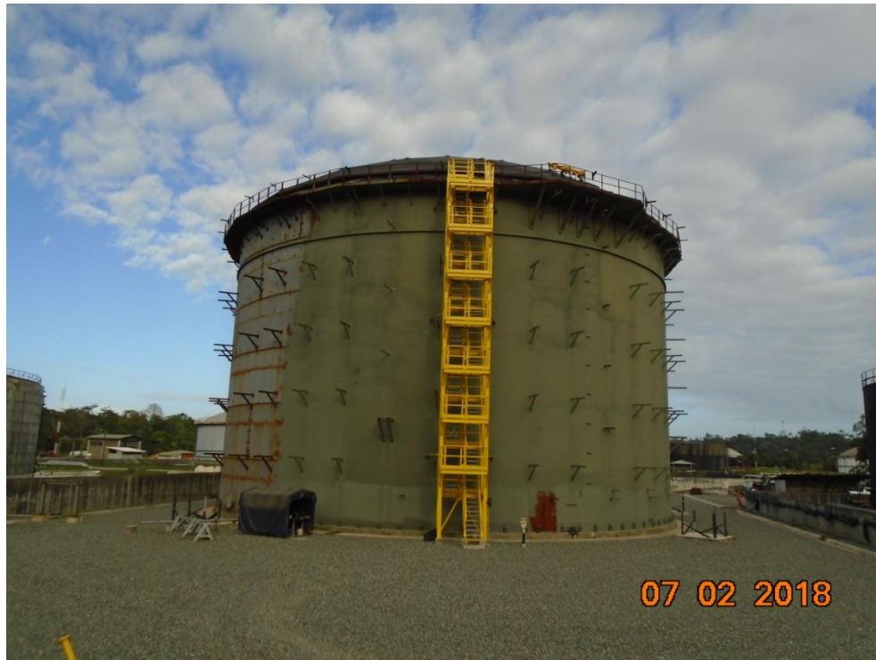
Tanque Bunker YT-7212
