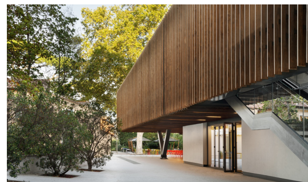
Figura 53. Fuente: Archdaily, Campus Hub.
