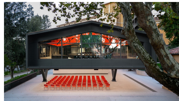
Figura 52. Fuente: Archdaily, Campus Hub.
