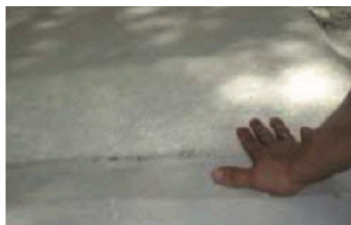
AFTER: By grinding down the sidewalk, the risk of a trip and fall is greatly reduced.
