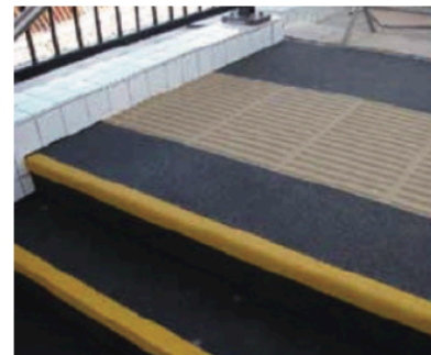
If stairs in your facility don't have good slip resistant properties, it may be possible to retrofit the stairs to achieve significant improvements. "SlipGrip Stair Tread Covers" is one example of a product that provides a rough surface on each stair tread to give people more traction.
