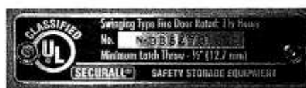
Figure 5-12 An approved fire door has a label indicating its classification and rating.
